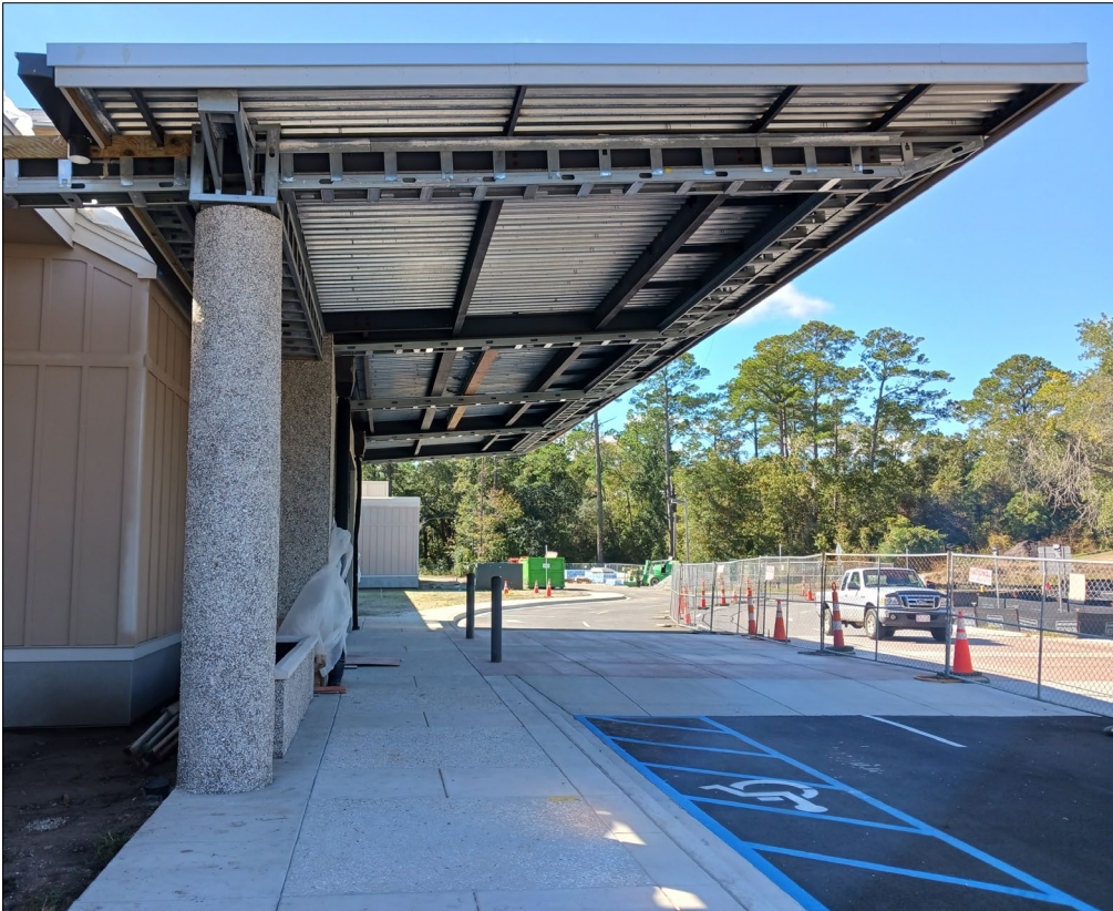
FRONT EXTERIOR VIEW
